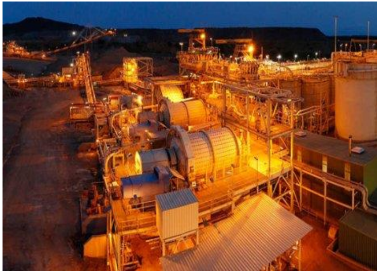
Teranga, Sambola, Senegal Processing Plant (Day and Night Views) www.google/image-indianmart.com Figure 1.4
